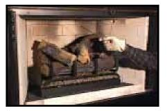
Figure 16 - Checking for Spillage
